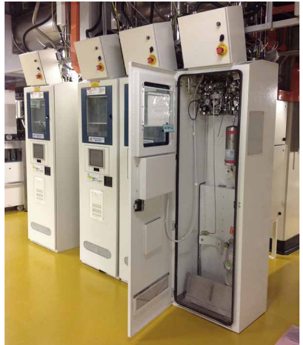
Photos showing CLEANVENT integrated in the supply panel within gas cabinets
